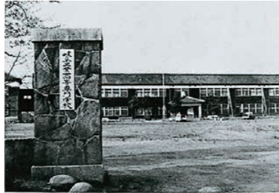
Unuma Temporary School Building (1963)
