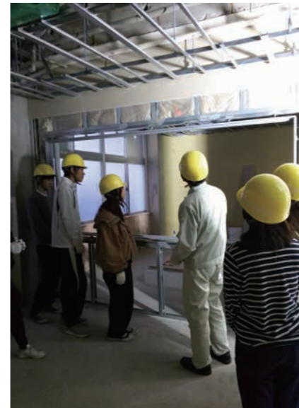
Observation of the building during construction
